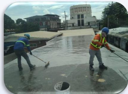
**“Single component, hand applied, Aliphatic waterproofing membrane”**
