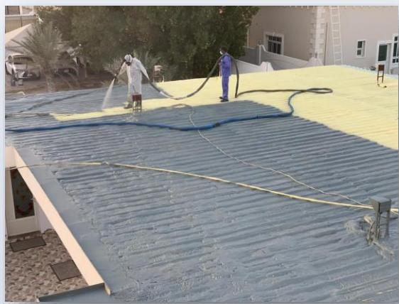
**“Two component, spray applied, seamless, general-purpose protective Coating”**
